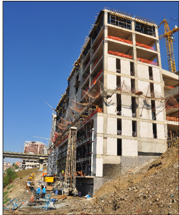
Fig.4. General view of drilling stage
